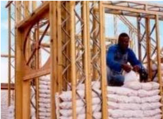
Fig. 3.9: The Eco-Beam and sandbag system by engineer Mike Tremeer ([earthbagbuilding.com/articles/eco-beam.htm](http://earthbagbuilding.com/articles/eco-beam.htm))
